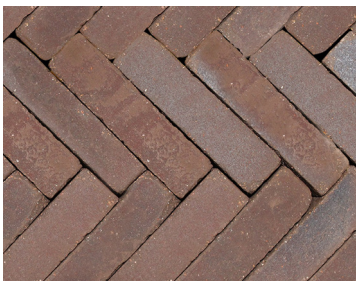
Gebakken klinker in keeperverband
