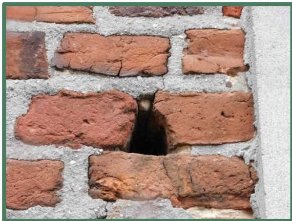
Foto 14: Opening in de gevel.
